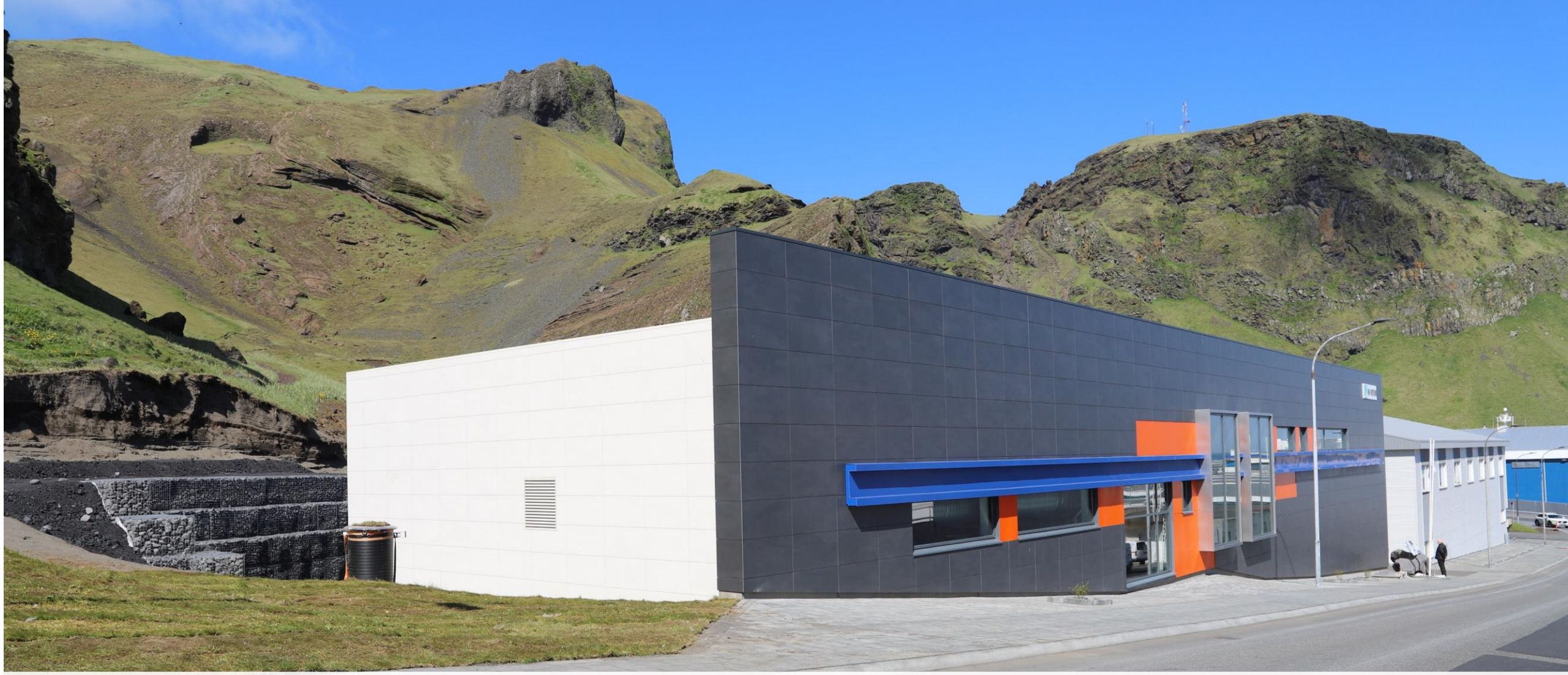
Sea Water Heat Pump Station
