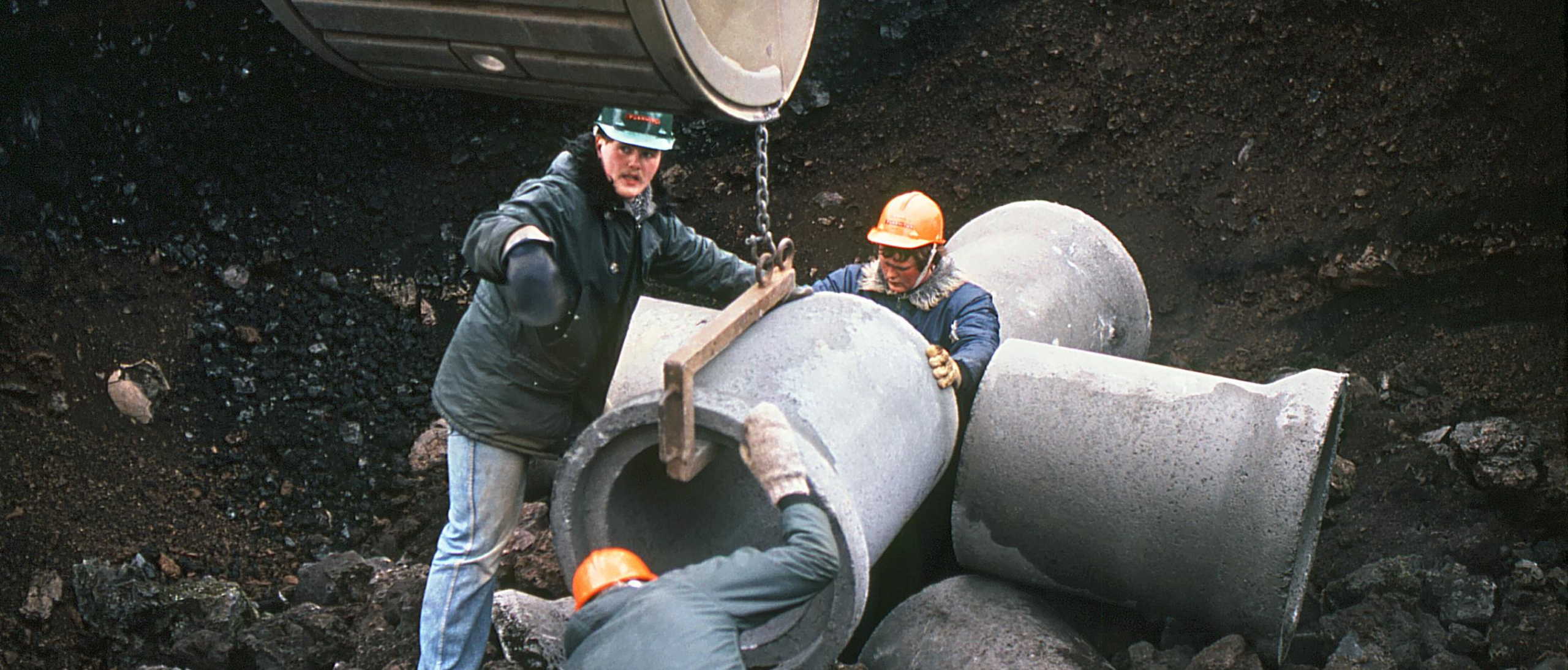
Steam collector installation
