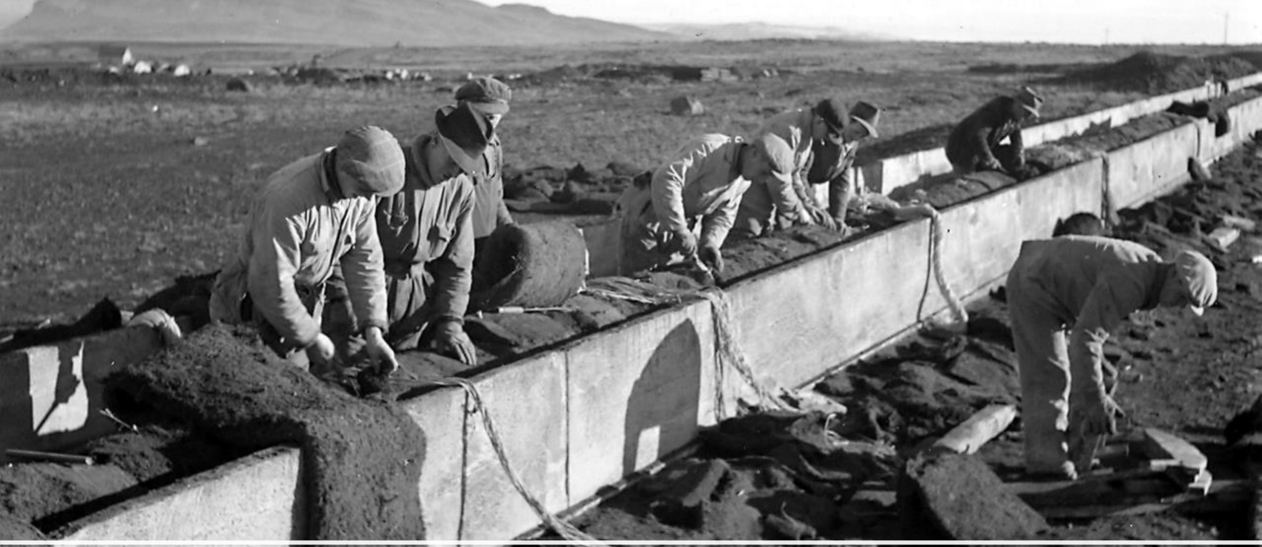
Pipe insulation with Icelandic turf
